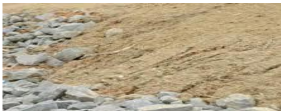
Fig. 16. Stone protective coating used to stabilize sand dunes [27].
